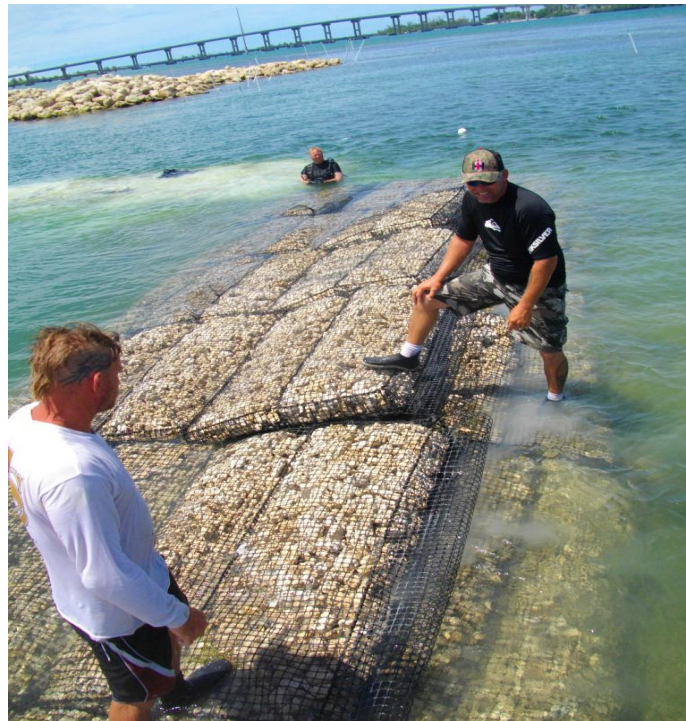
Figure 9. Marine mattress on filled geotextile tubes
